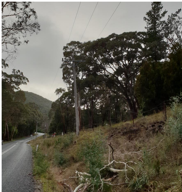
Fire start on REFCL protected feeder 4 th July 2018, Mt Macedon – tree taking out single phase
